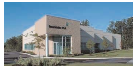
Building of CCL, CLT (Center for Laser Technology), and Fraunhofer USA Headquarters in Plymouth, Michigan
